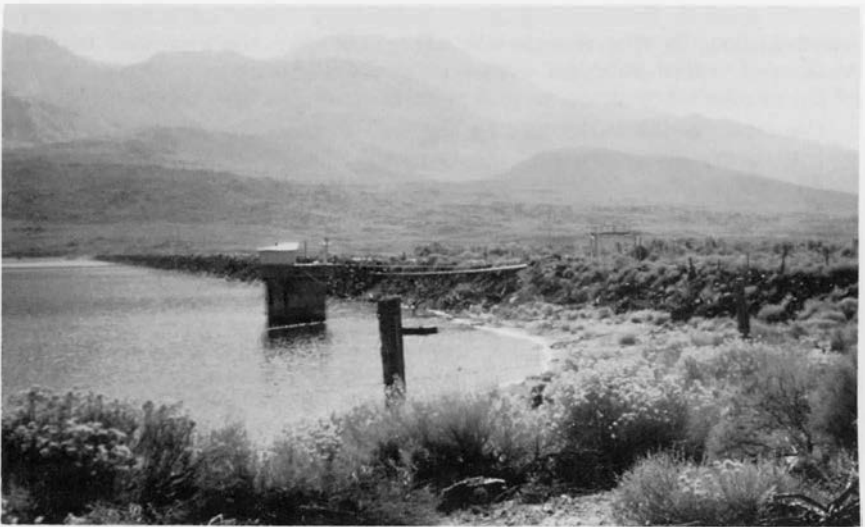
Tinemaha Dam in Owens Valley, built with mules rented from Bev Hunter pulling the old Fresno scrapers. Photo by Lester Reed in 1965.
